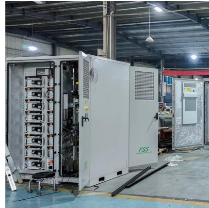
30kW Off-Grid Solar System
