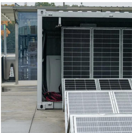
Energy storage container, BESS container
