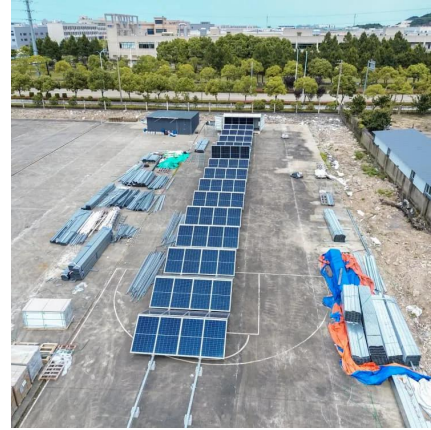
Colombia: 2MWh LFP battery storage unit in to go online soon
