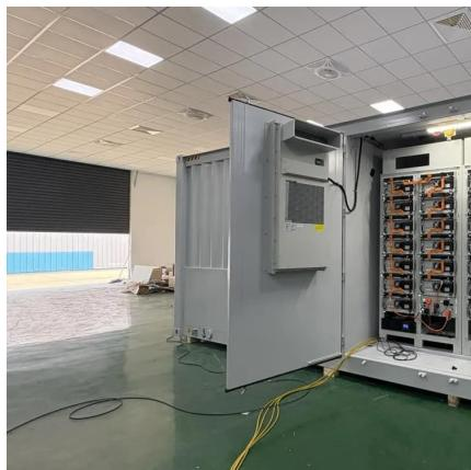
[Containerized Battery Energy Storage Systems \(BESS\)](#)
