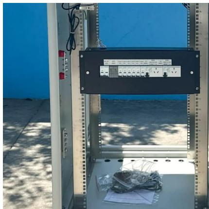
[Assembly for \(1\) Rack PDP solution UPS & Ext. Battery, ...](#)
