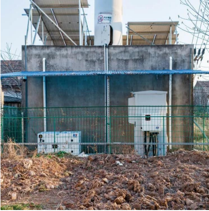
El Salvador battery container storage
