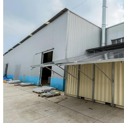
Battery Energy Storage Containers: Mobile ...
