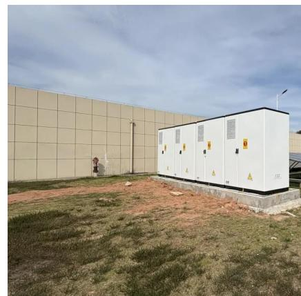
[Containerized Battery Energy Storage Systems \(BESS\)](#)
