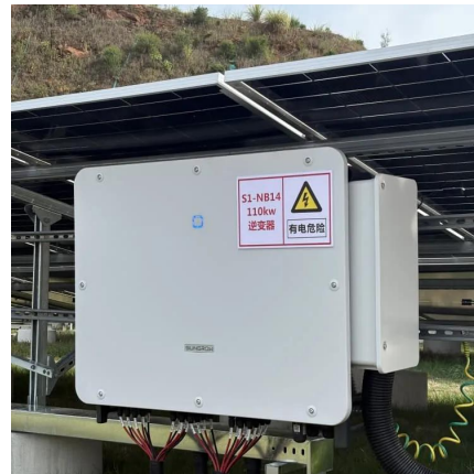
Top Off Grid Inverters Suppliers in Nicaragua
