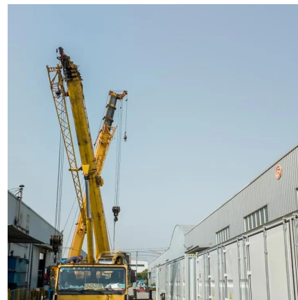
CATL's TENER Stack: 9 MWh Containerized Stacked BESS ...
