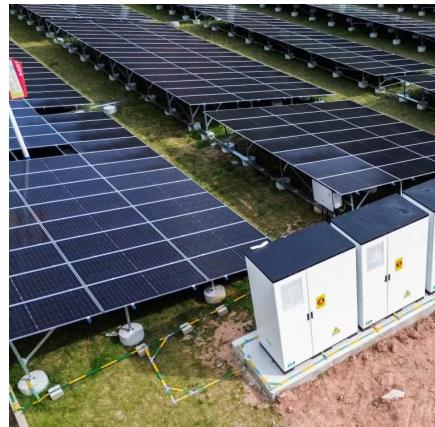
[Lithium iron phosphate battery energy storage container](#)
