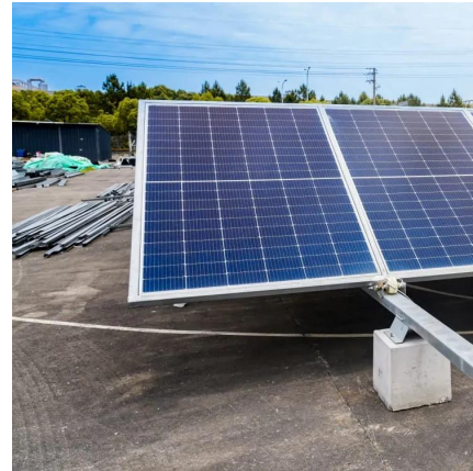
How to Install Solar Panels on a Roof: A Step ...
