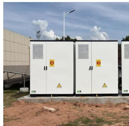
[Containerized Battery Energy Storage Systems \(BESS\)](#)
