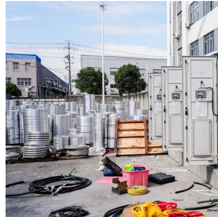
Communication container station
