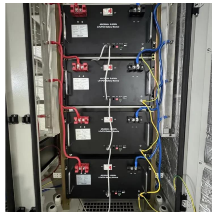
How to Assemble a LiFePO4 Lithium Battery Pack for Solar ...
