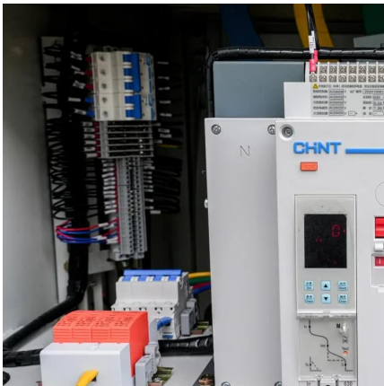
Rezolv Energy breaks ground on one of biggest solar power ...
