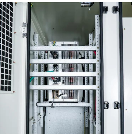
SIMOPRIME Medium-Voltage Switchgear
