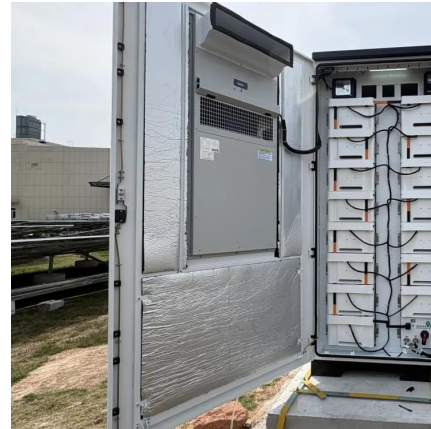
Cabinet Energy Storage System , VREMT
