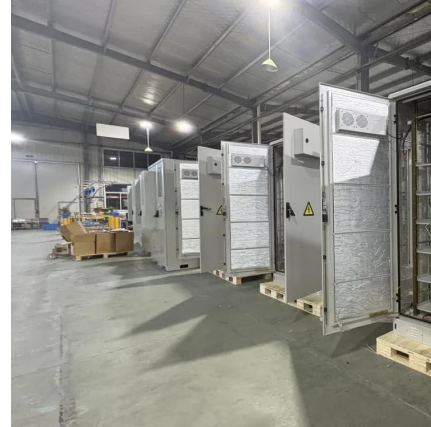
Mobile energy storage site inverter grid-connected 4g ...
